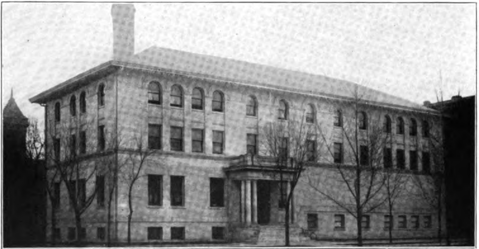
Y. M. C. A. BUILDING, HASTINGS
