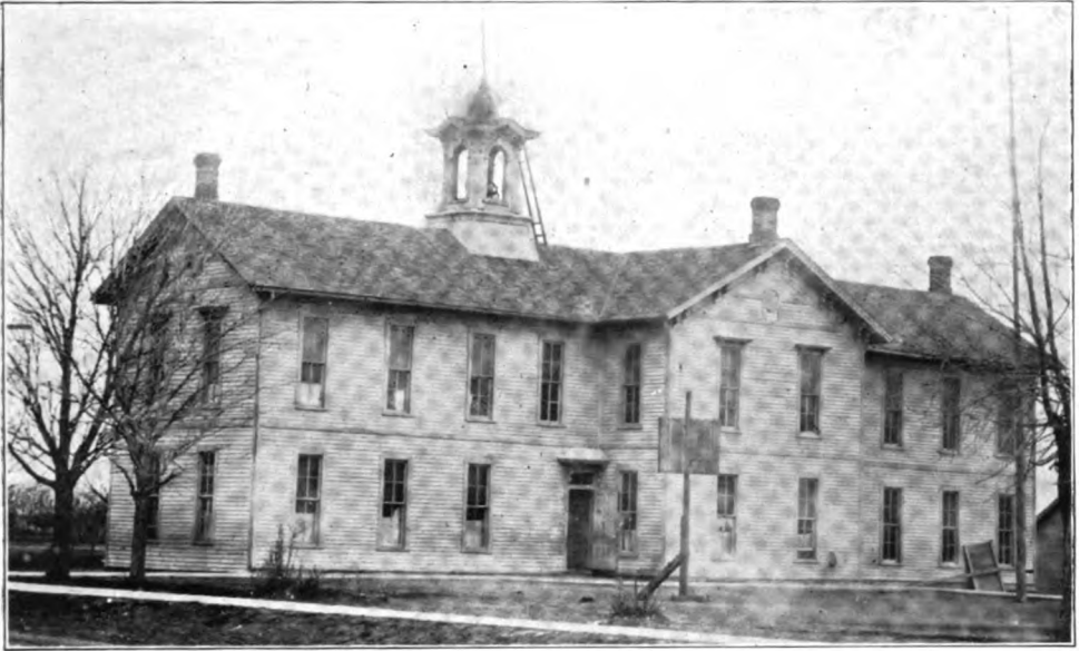
OLD PUBLIC SCHOOL BUILDING, JUNIATA
